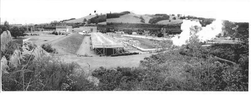
This composite picture of the Wairakei Geothermal Power station shows the binary plant in the foreground with the two power stations beyond with thire switching yards on the far left. The prawn farm ponds are behind the clouds of steam. To the right of the binary plant can be seen the pipes from the steam fields.
